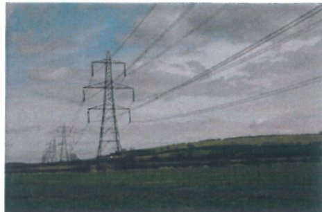
THE PYLON LINE PROPOSED THROUGH THE COUNTRYSIDE
